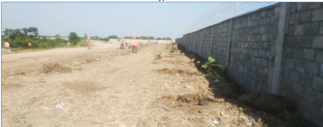
Plantation at STP front side compound wall
