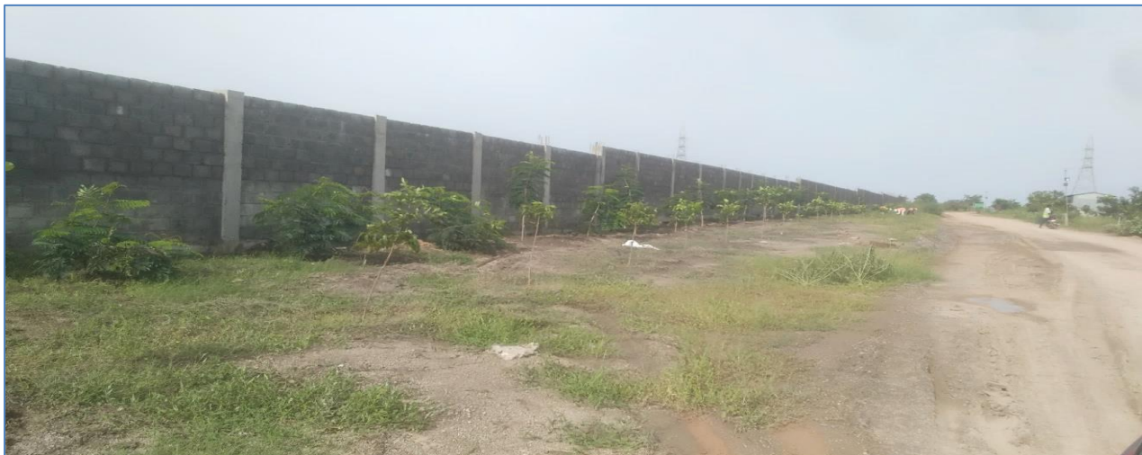
Main gate to Old OHC compound wall - Before
