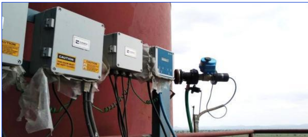
PM CEMS for Cement Mill Bag House Stack
