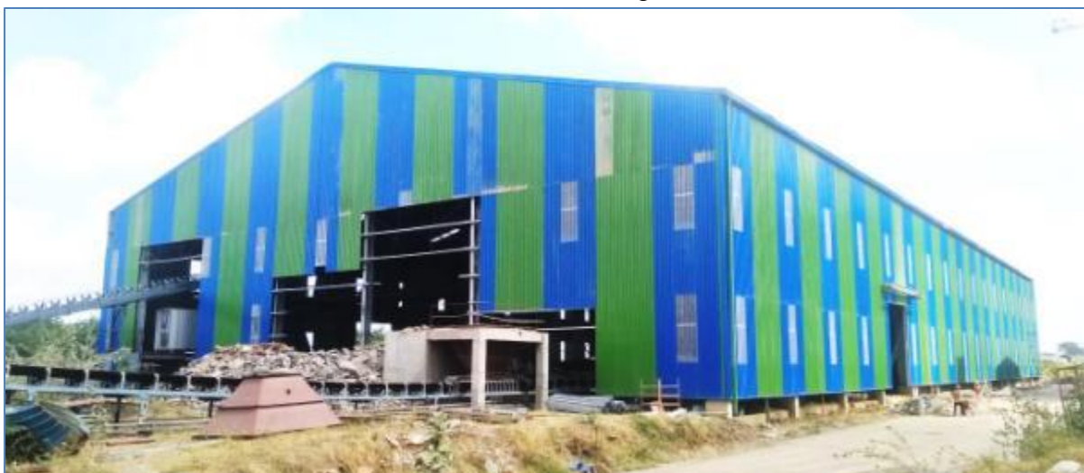
Closed Additive Storage Shed
