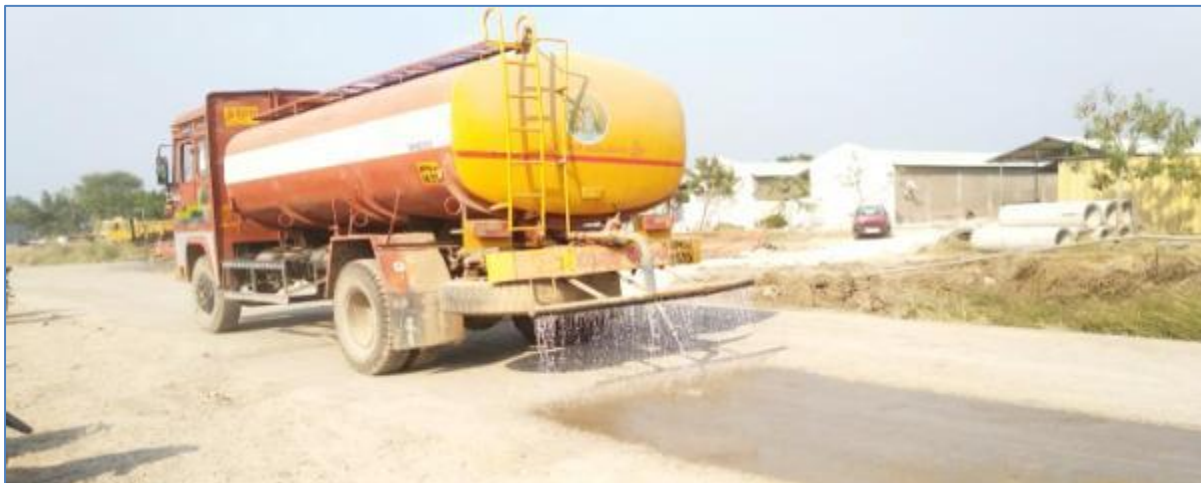
Water spraying through tankers on internal roads
