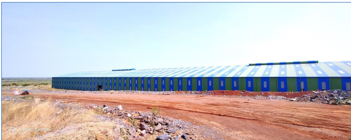
Closed Limestone Storage Shed
