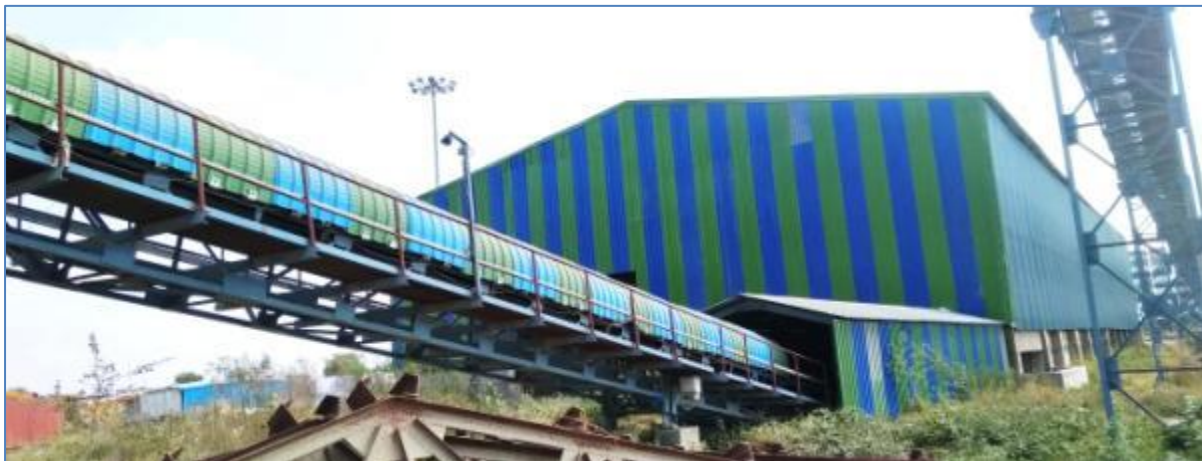
Gypsum storage shed & Closed conveying system
