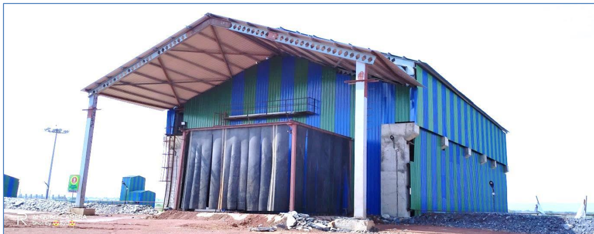
Closed crusher building and Dump hopper provided with rubber curtains
