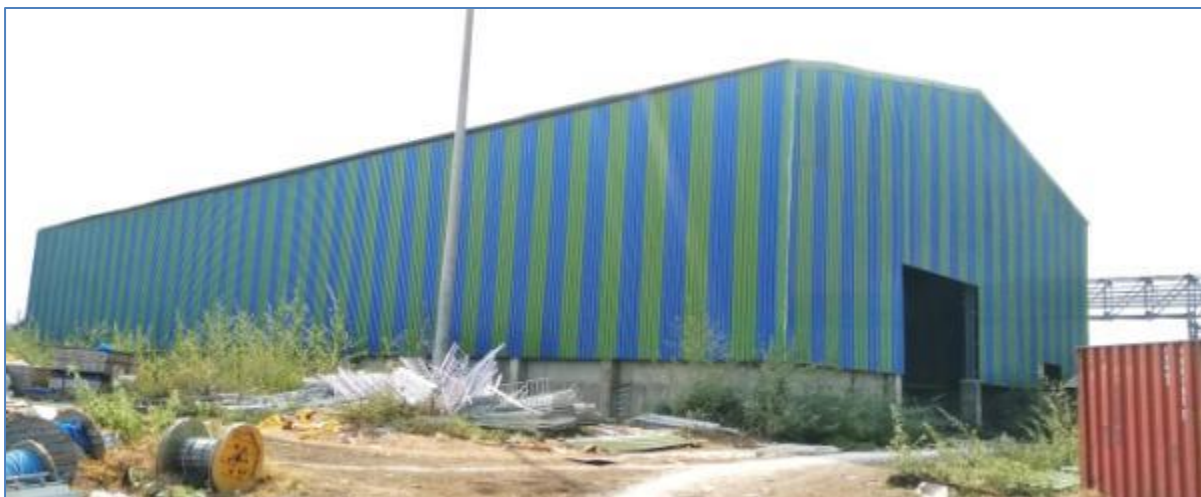
Closed Gypsum Storage Shed
