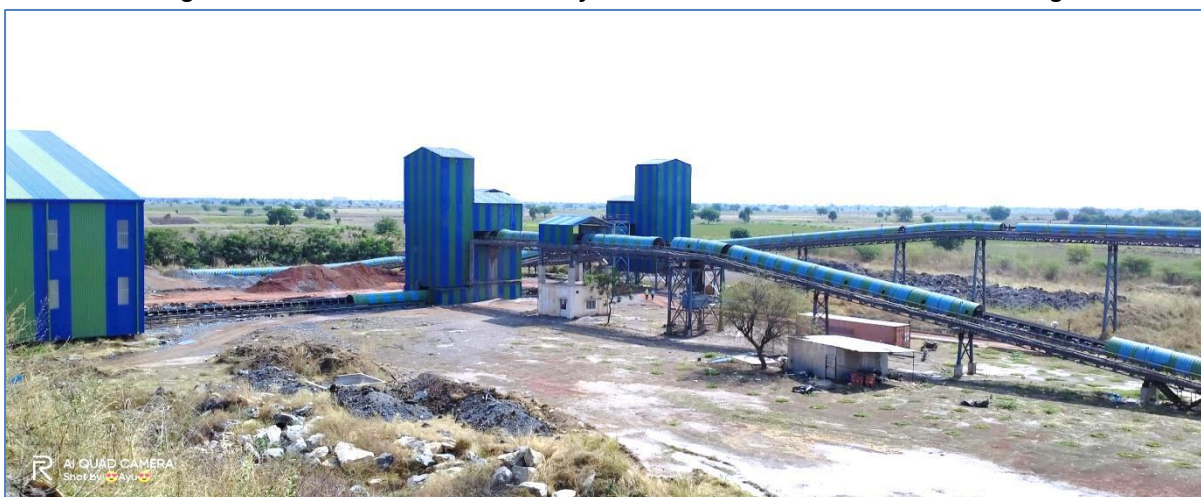
Closed limestone conveying system circuit
