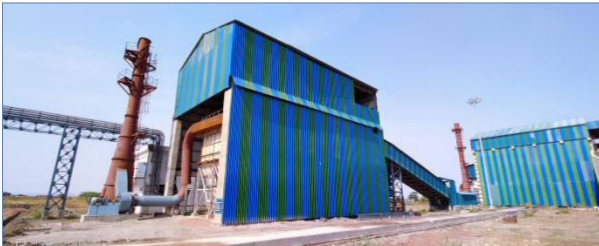
Bag Filter at Limestone Secondary crusher and closed crusher building
