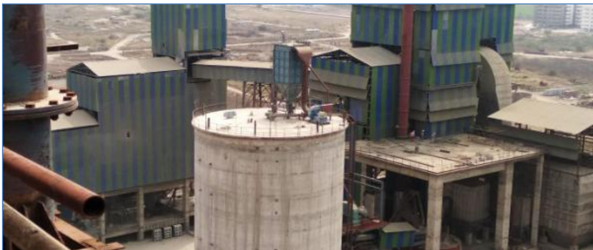
Bag Filters at Fly ash silo Top
